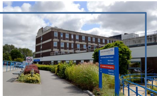
North Devon District Hospital (Barnstaple)
